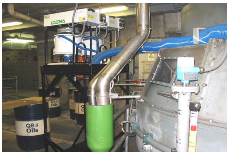
DARWIN D600 WITH SYNTESIS PRE FILTER ON ENERGY PLANT
